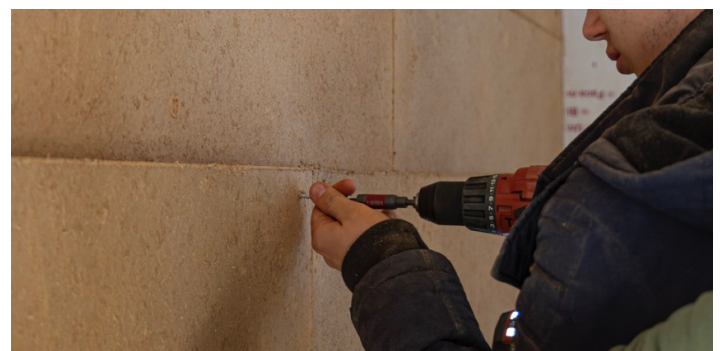
Figure 5 – Fastening the clay building board in our HDU
