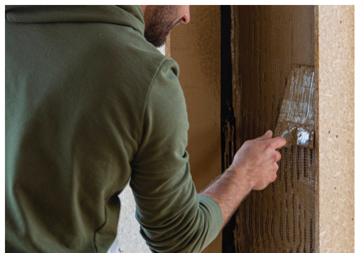
Figure 6 – Putting clay plaster on the building boards
