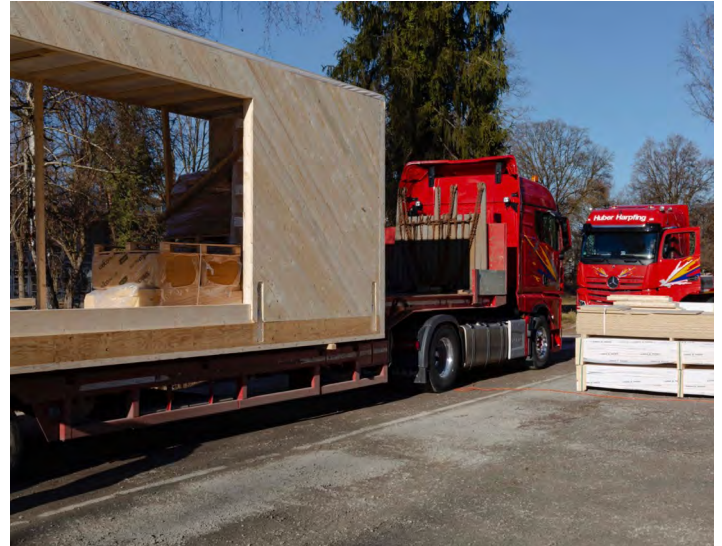
Figure 35 – Delivery of the wooden modules to the construction site
