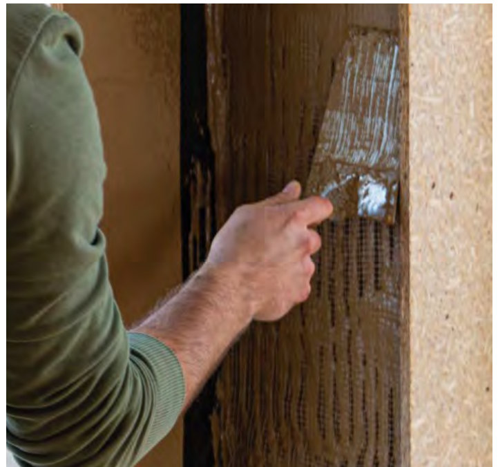
Figure 41 – Clay plaster on the clay building boards
