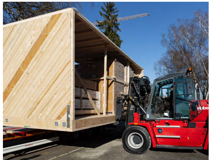
Figure 36 – Unloading the modules with a forklift
