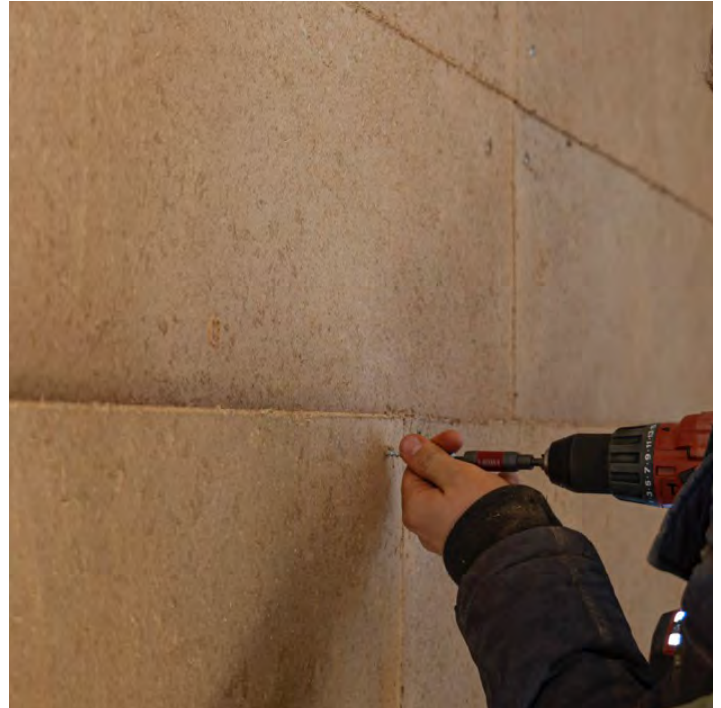
Figure 40 – Fastening the clay building panels in the interior
