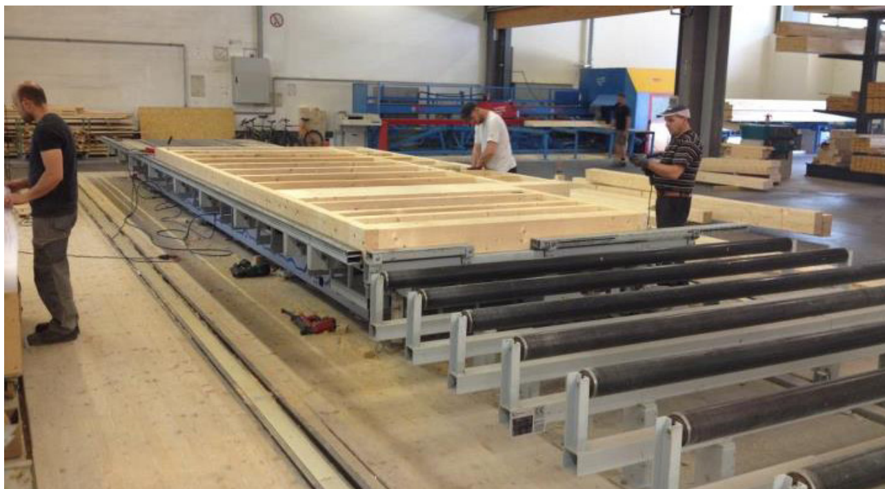
Wall prefabrication at Rubner Haus, Bozen
