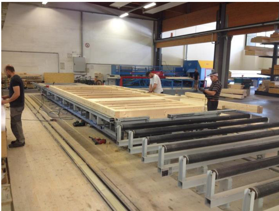
Wall prefabrication at Rubner Haus, Bozen
