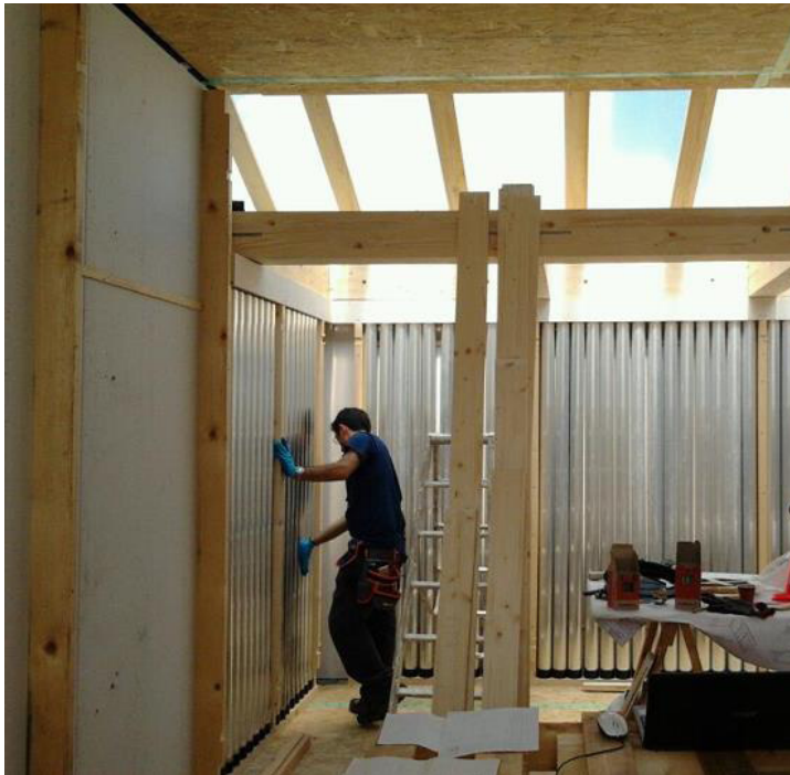
Cavity in the wall with sand
