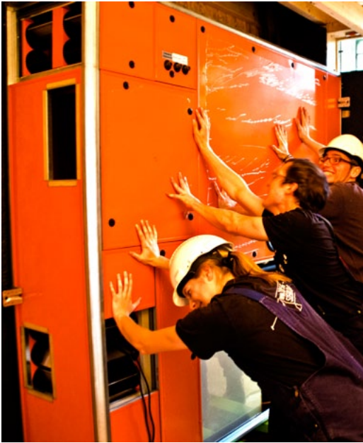
Installation of the Air Handling Unit
