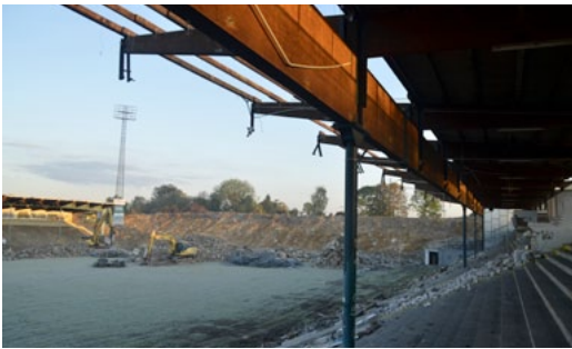
During the demolition of the "Tivoli"
