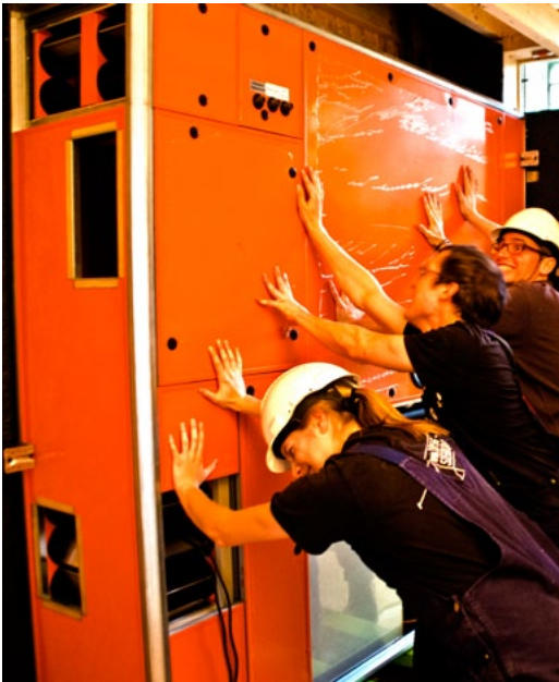
Installation of the Air Handling Unit
