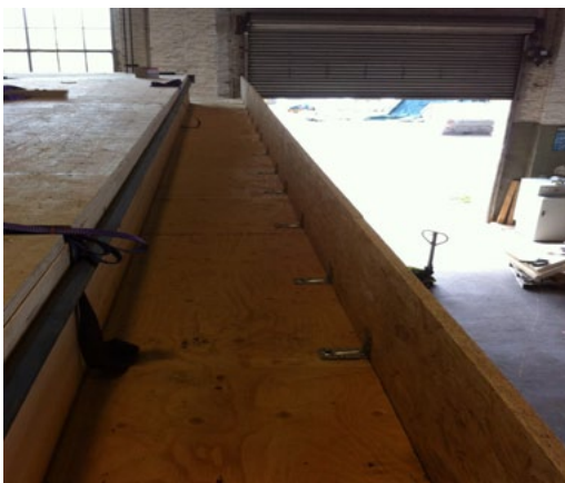
steel band and gutter
