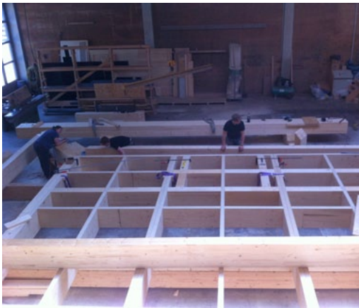
beams inside the roof
