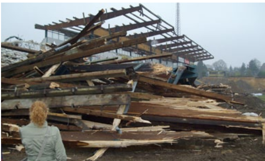
The "Tivoli" beams after the demolition
