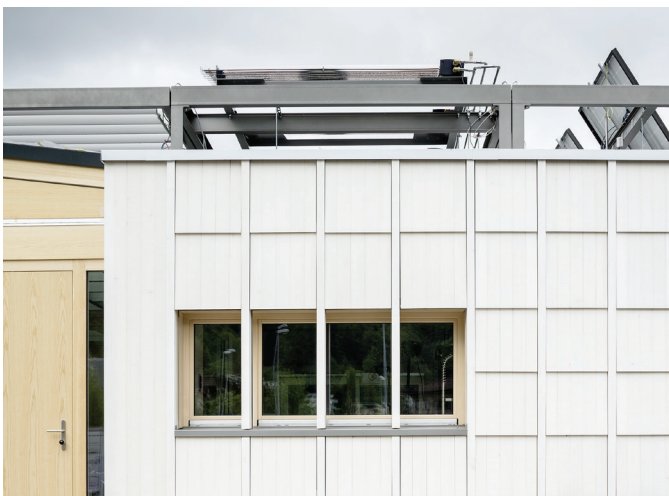
Img. 21 Window south kitchen
