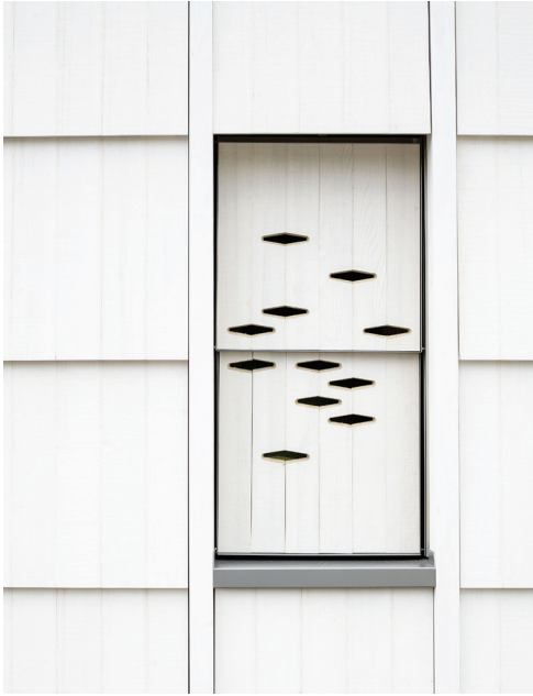
Img. 10 Shading shutter down
