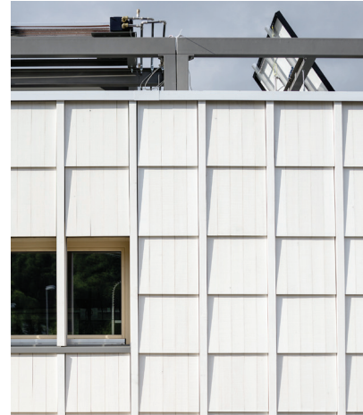
Img. 9 Example of the wooden facade
