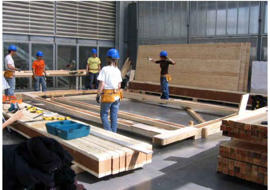
Photos 6. SKIN - Views of STEICO portal frames under construction with at GAIA SKIN - Enveloppe isolante. Vues des portiques STEICO en cours de construction aux GAIA
