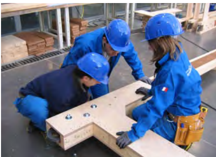
Photos 6. SKIN - Views of STEICO portal frames under construction with at GAIA SKIN - Enveloppe isolante. Vues des portiques STEICO en cours de construction aux GAIA
