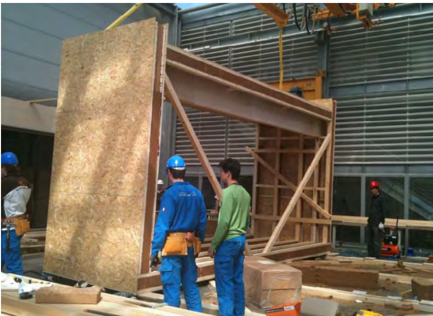
Photos 7. SKIN - Views of timber boxes under construction with at GAIA SKIN - Enveloppe isolante. Vue des anneaux en cours de construction aux GAIA
