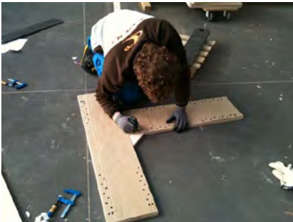
Photos 6. SKIN - Views of STEICO portal frames under construction with at GAIA SKIN - Enveloppe isolante. Vues des portiques STEICO en cours de construction aux GAIA
