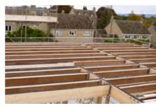
STEICOjoists fulfil the demands from house builders for greater clear spans and better dimensional stability, whilst not increasing the size of the cross section of the construction elements. STEICOjoists have a high strength to weight ratio in relation to its equivalent solid
