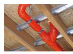
The amount of pipes for plumbing and air conditioning in modern buildings is growing constantly. Installation of services on the intermediate floors can cause problems and can lead to unnecessarily deep floor build ups and increasing costs. Using the STEICOjoist you can drill certain service access
