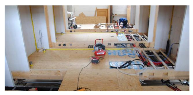
Figure 9: Pipelines in the floor already build
