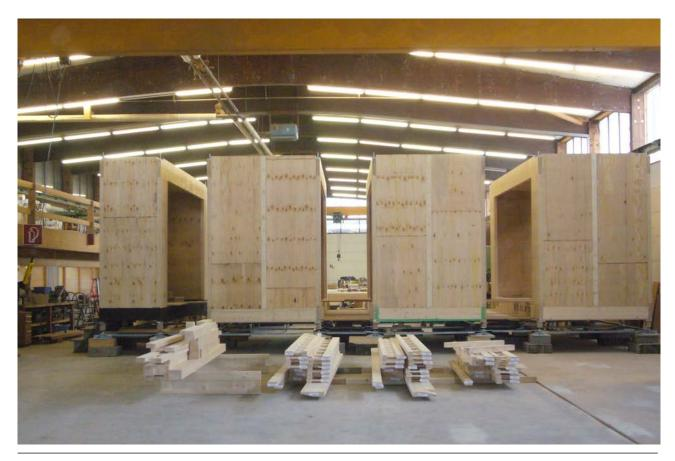
The next day is reservated for the gaps and the tower. the floor of the gaps are the first assembled elements. The tower and the vertical parts of the gaps are prefabricated too and have to be assembled with the use of a crane. Special attention is necessary because of the high use of glazing.
