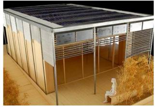
Rather than opting for the popular box and panel design, the unique-looking Fablabhouse from Instituto de Arquitectura Avanzada de Cataluña is shaped for optimum solar capture and incorporates photovoltaic imprinted textiles on a ribcage of reinforced bars.
