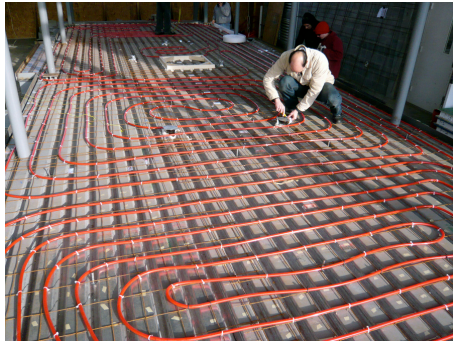
Setting the radiant floor and polishing the concrete slab
