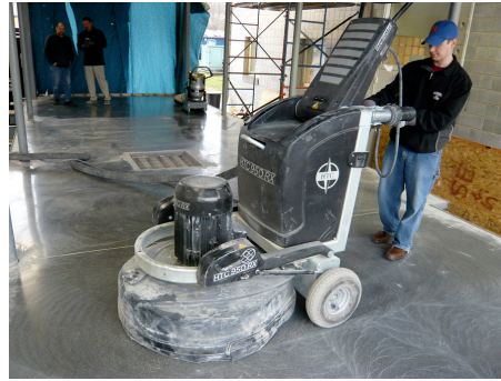
Setting the radiant floor and polishing the concrete slab
