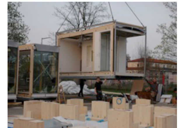
The first module is placed on the foundations for test assembly.
